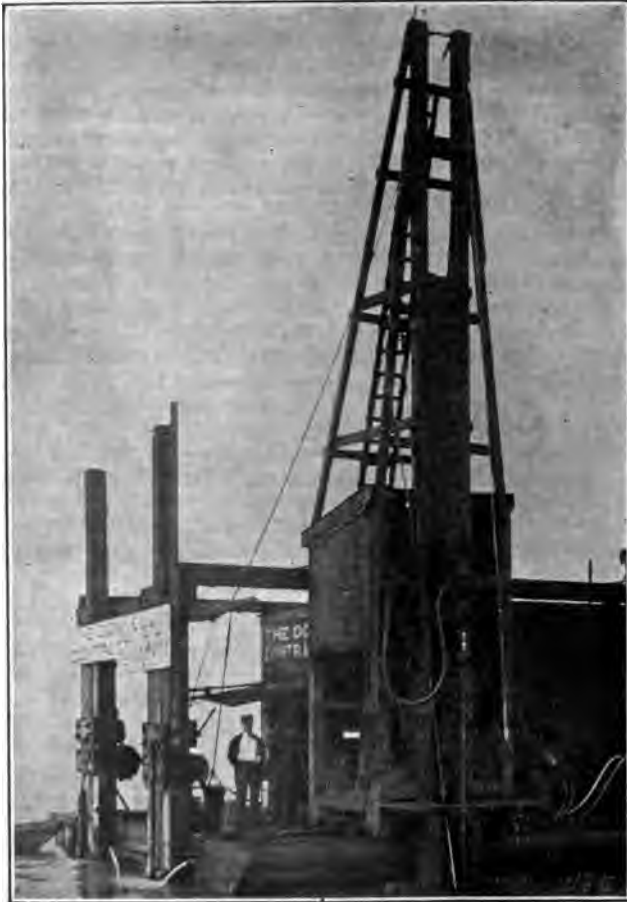
Fig. 172. Drill Frame on a Drill Boat.
